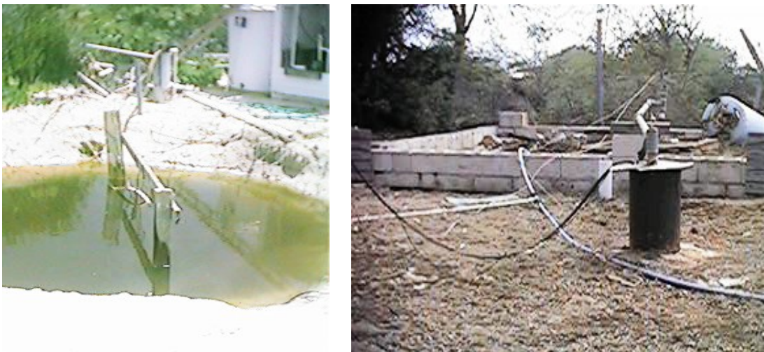
Figure 11 Example of private water well (left) and pumping station for Codrington (right)
